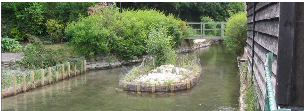
Green revetments to bank and island
