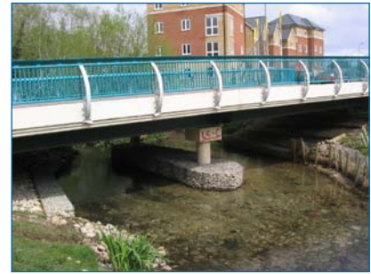
Letcombe Park revetment work
