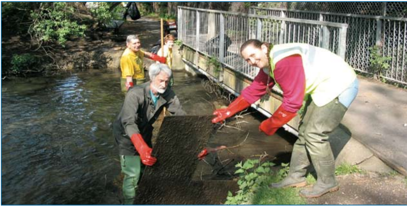
Local people clear out 5 skips of rubbish from the brook.
