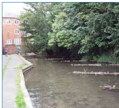
Wantage flood alleviation works
